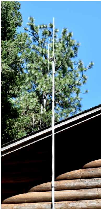
Antenna above Roof Line. Antenna is attached to a securely mounted pole. Try to avoid objects (e.g., branches, etc...) being within 10 to 15 feet of Antenna (for better propagation).
